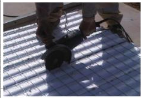
Test on polystyrene wall Fig. 6. Cutting of panels
