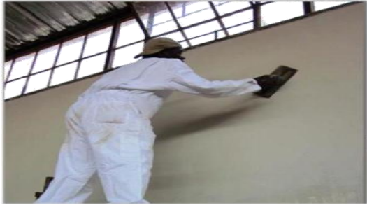
Fig. 5. Finishing of last layer
