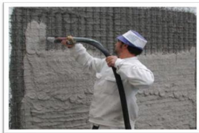
Fig. 4. shotcrete by machine
