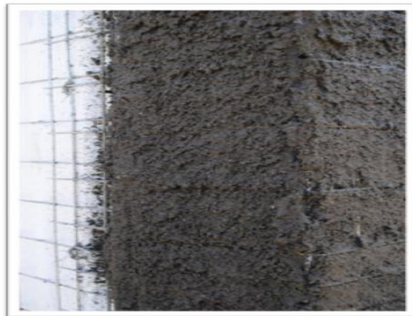
Fig ,3. First layer of plastering
