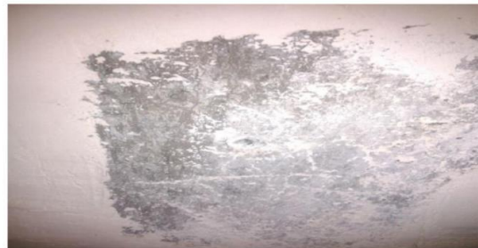
Fig. 9. Bullet test do not penetrate inste just caused a minor dent Sound proof test
