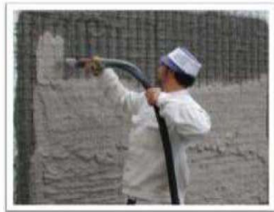
Fig. 5 Shotcrete by Machine
