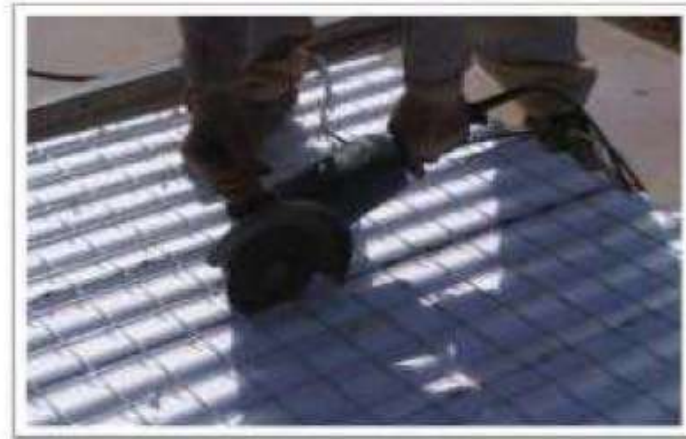
Fig. 7 Cutting of Panels
