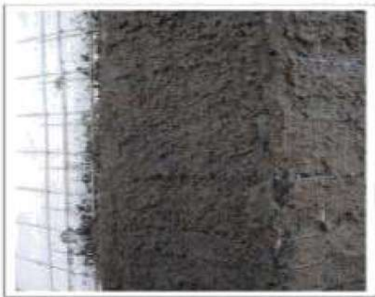
Fig. 4 First layer of plastering
