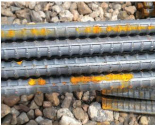
Figure 1 – Light rust on the bar is acceptable.
