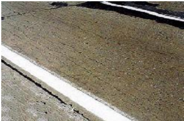
Figure 12 Alkali-aggregate reaction
