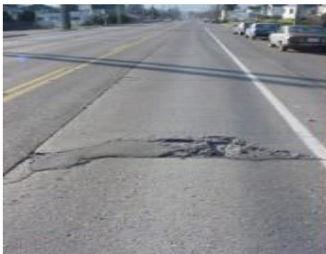
Figure 4 Spalling
