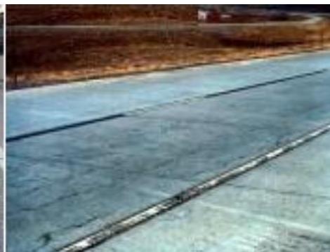
Figure 5 Shrinkage cracks
