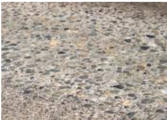
Figure 6 Polished aggregates
