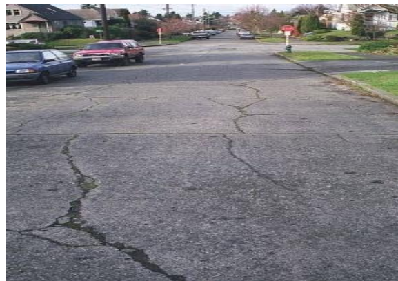
Figure 9 Linear cracking
