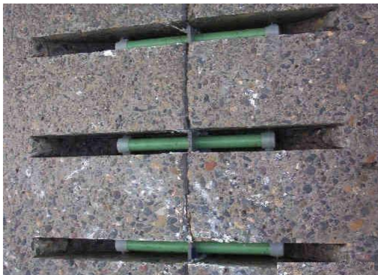
Figure 17 Dowel bar retrofitting
