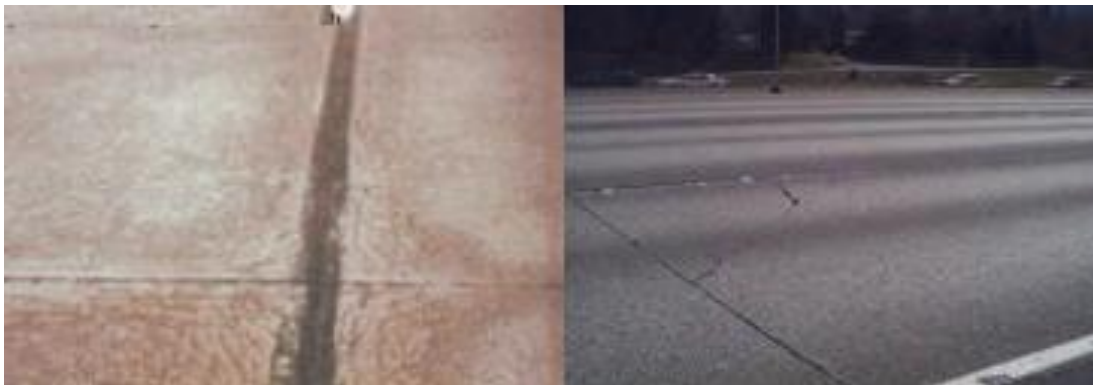
Figure 10 "D" cracking
