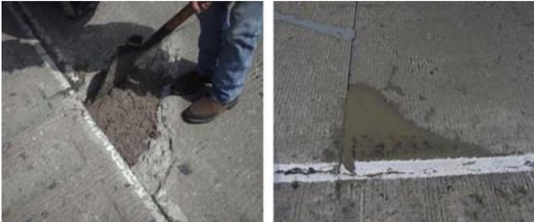
Figure 16 Patch repair
