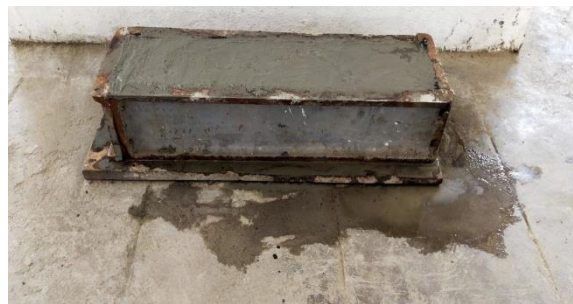
Fig 4.2 Casting of specimens
