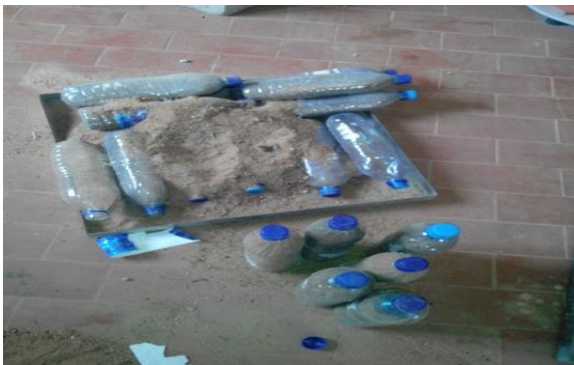
Plate1: bottle bricks after filling
