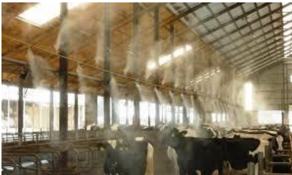
Fig 3 Fogger System in Livestock Shed
