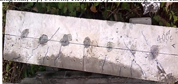
Fig.2.6 Beam crack pattern at 400°C after repair with repair material 1
