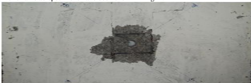
Fig. 3 First crack of mild steel reinforced slab
