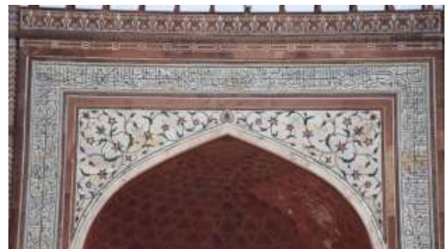
Fig. 6 – Spandrels of the arched entrance gate to the Taj Mahal
