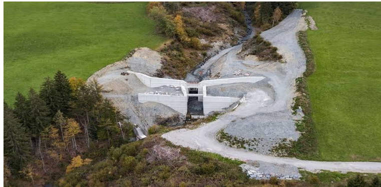
CONCRETE CHECK DAM
