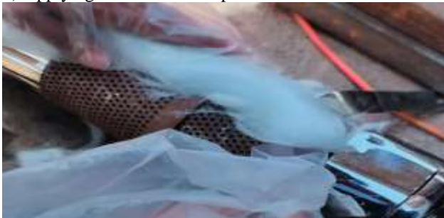
Fig.13. Applying Glass-wool .
