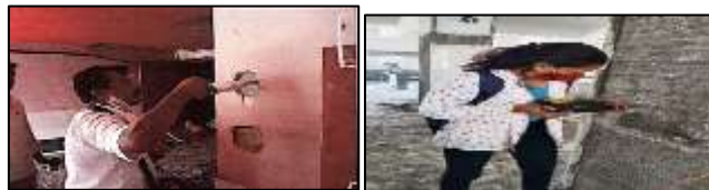
Figure 2: Rebound Hammer Test before jacketing Figure 3: Rebound Hammer Test after jacketing
