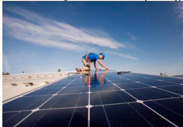
Figure 2 A person cleaning PV panels manually [16]
