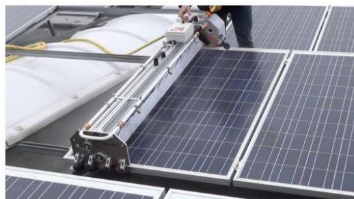
Figure 14An example of a 'Wash Panel' system
