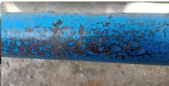
Photo showing clean water supply pipeline in the water supply pipeline in company after treatment with scrubbing paste.
