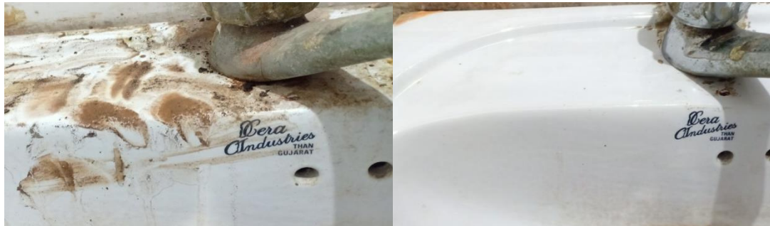
photo-rust stains on wash basin
