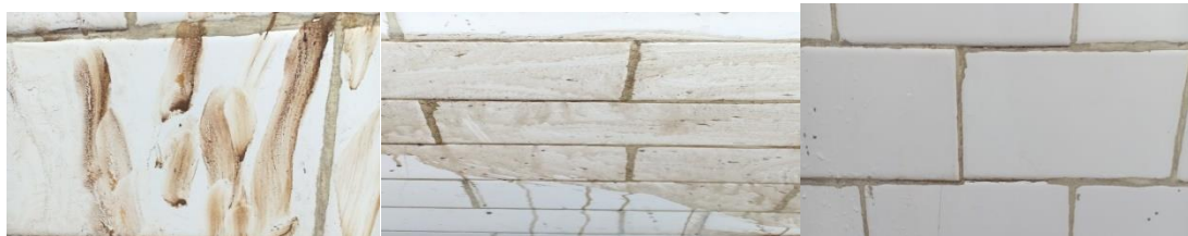
Photos(a) rust stains on vitrified tiles (b)during suspension wash (c) Clean bathroom tiles.
