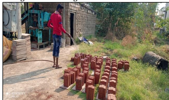
Figure 3.4: Curing of Laterite Bricks
