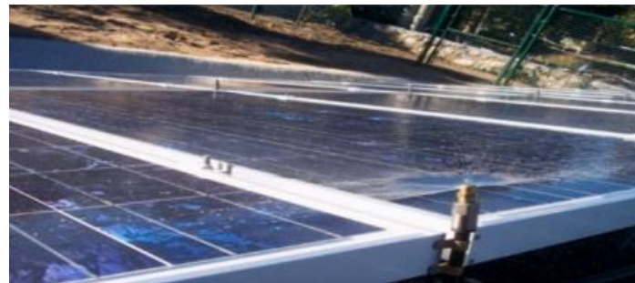
Fig7: Heliotex cleaning system
