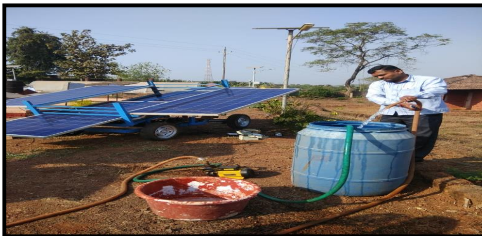
1 Pictorial view of water pump operating on portable solar photovoltaic power system
