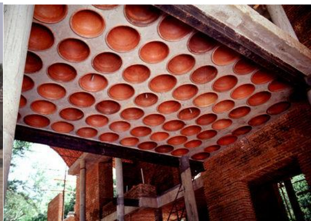
Fig 9. (Right) - Filler slab
