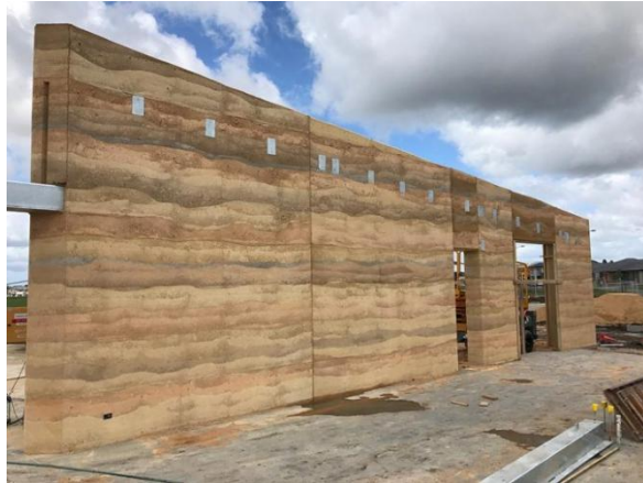
Fig 7. Rammed earth wall.
