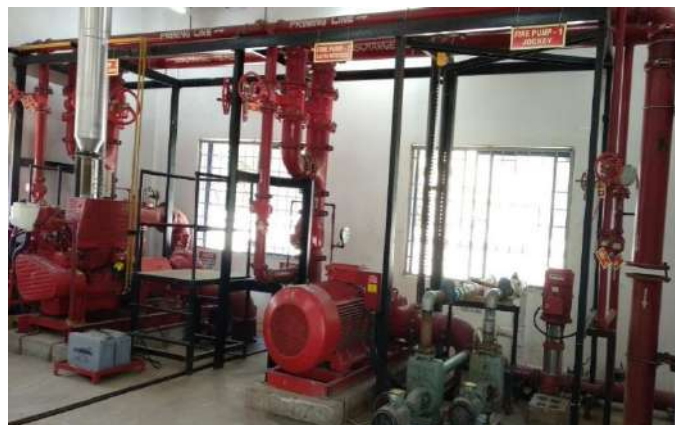
Figure 3.4 Fire pumps- Main (Diesel), Electrical, Jockey pumps
