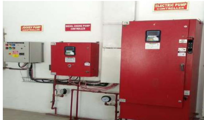
Figure 3.2 Fire pumps Control Panels
