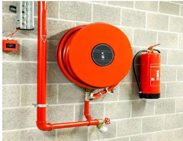
Figure 5.8 Fire hose reel
