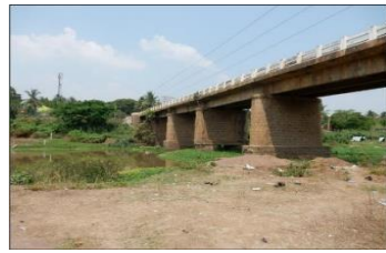
Fig 1. Image of bridge
