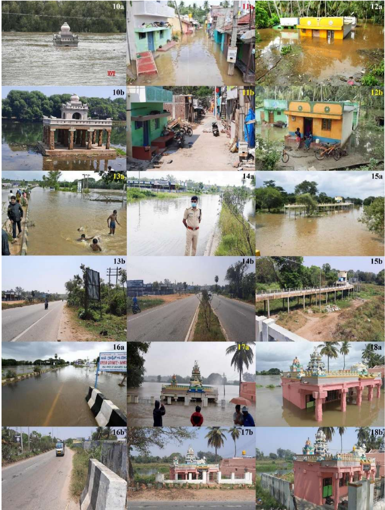
Plate-II: (a) During and (b) After the Flashflood impacts of Kapila River on 10. 16 Pillar tomb; 11 & 12. Streets near Main temple; 13. NH-712 near Mallanamoole Mutt; (i) Nanjangud Water works; (k & l) Road block of NH-766 from Mallanamoole Mutt till Mysore Paper Mills Kapila river water submergence (a, b, c d & e) Blocking the road between Mallanamoole Mutt to Mysore Paper Mills on NH-766; (f) Submergence of Parashurama Temple
