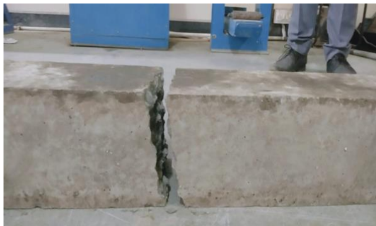
Fig 13: Beam After Fail
