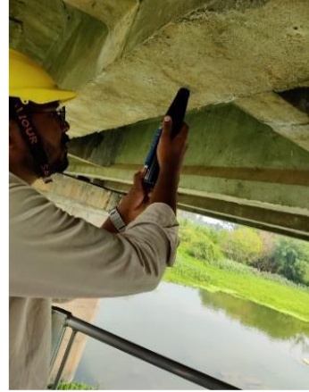
Fig 2: Rebound hammer test
