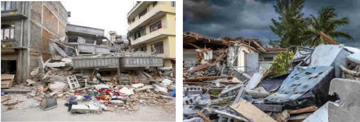
Fig. 3 Impact of earthquake
