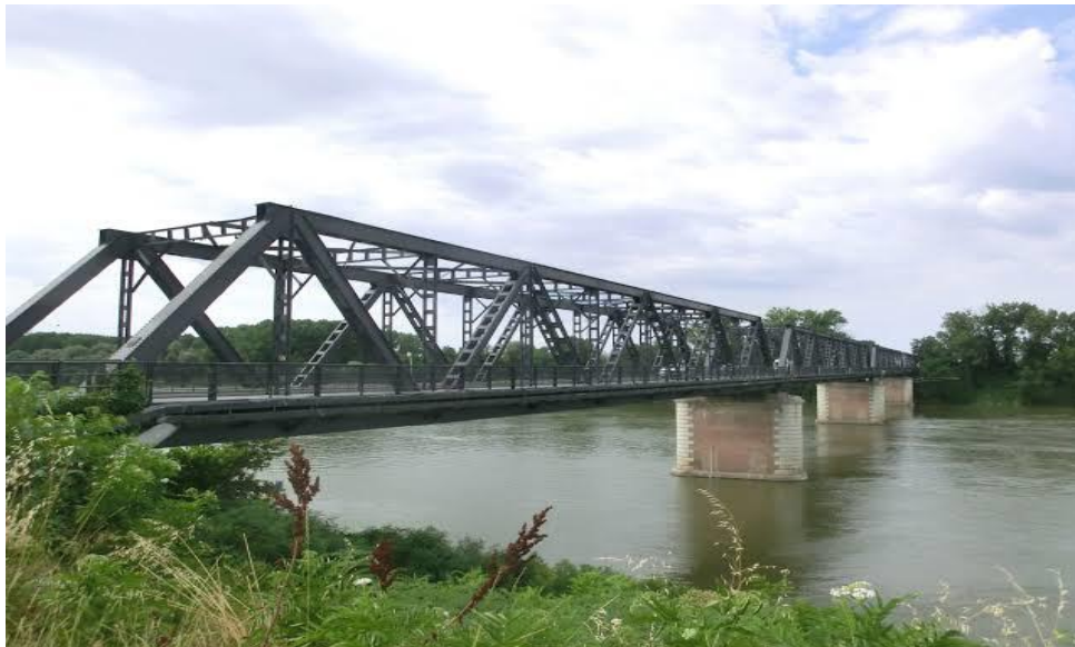
Fig. 12 Subdivided Warren truss bridge
