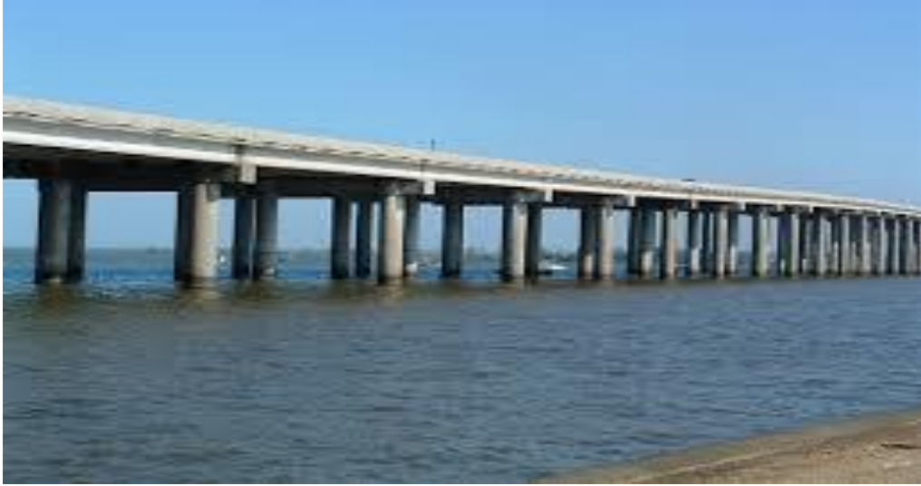
Fig. 11 Manchaca Swamp Bridge
