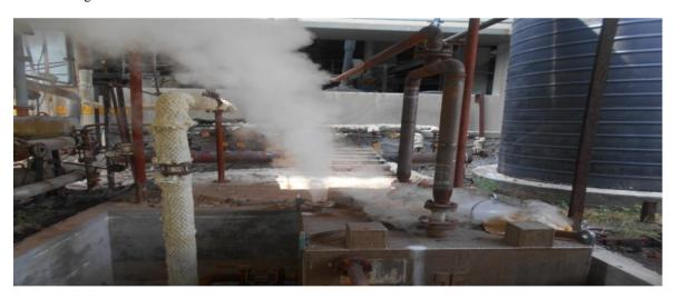
For flash steam recovery flash vessel will be connected and that flash steam will also heatthe feed water. As shown in fig
