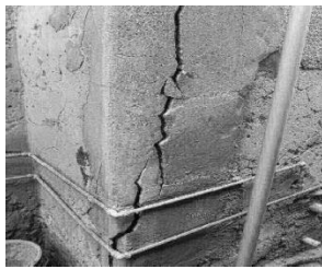
Structural cracks
