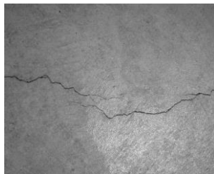
Non-Structural cracks
