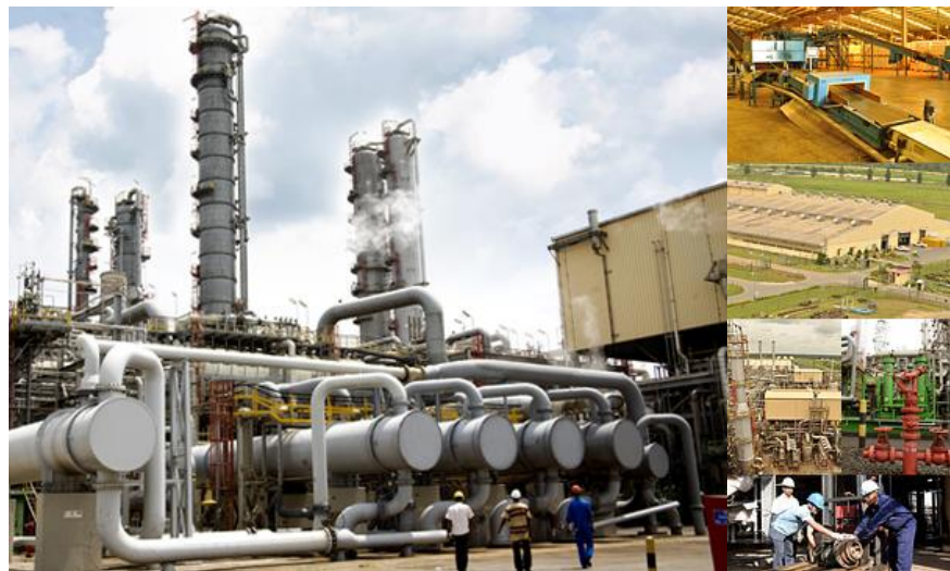
Fig 3: Indorama Eleme Petrochemical Plant
