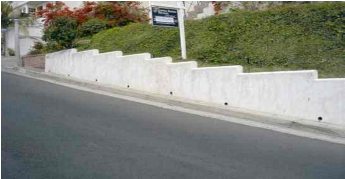
Figure 1.9 Concrete walls with weep-holes
