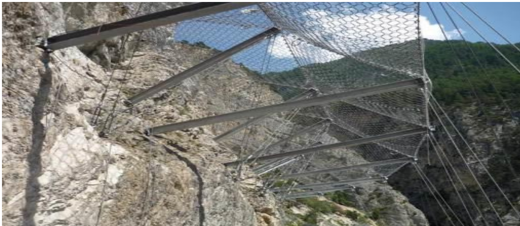
Figure 1.7 Mesh secured by bolts to arrest falling rock blocks
