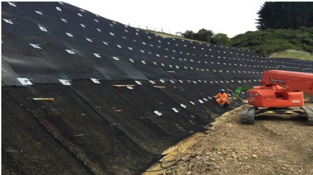
Figure 1.6 Slope protection work
