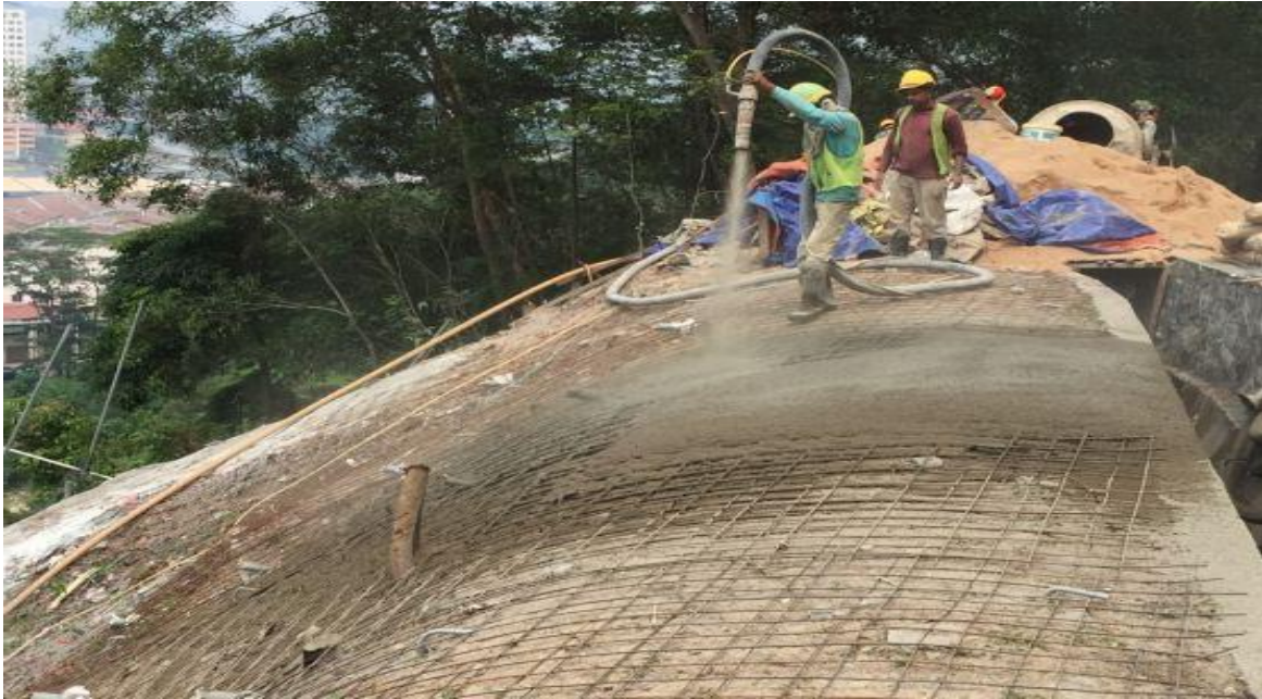
Figure 1.5 Shotcrete application in slope stabilization
