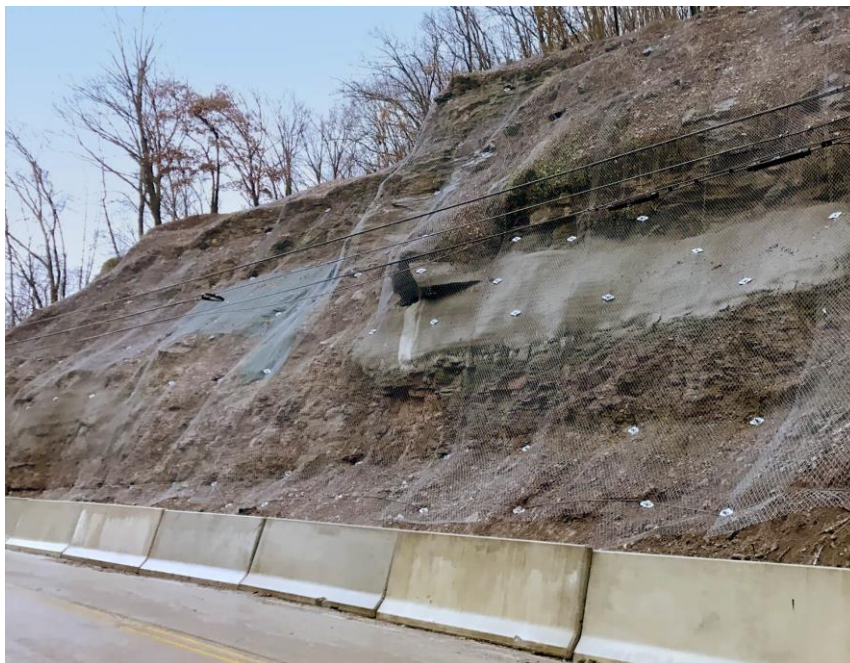
Figure 1.3 Rock bolting & wire mesh
