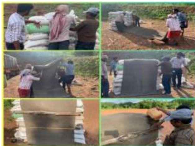
Fig3. Installation of Sentry post with Sand Bag
