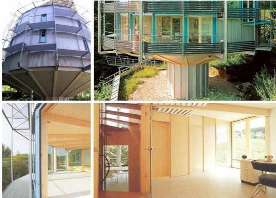
Figure 5. spinning solar powered house in german
