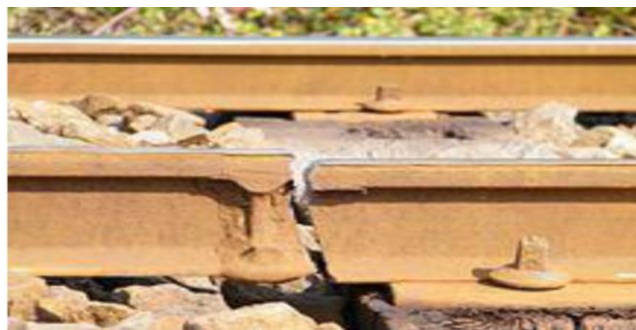
Figure 2 : Railway Track Crack [8]
