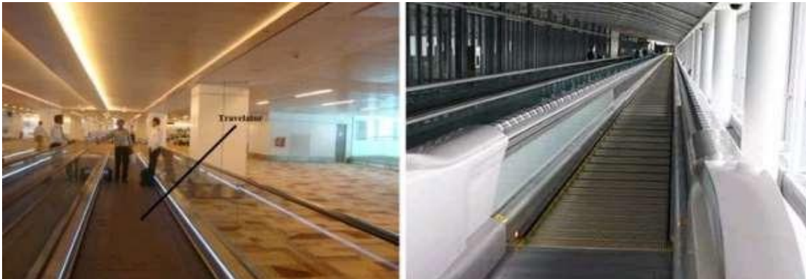
Figure 1. (a) Belt type moving walkway in Delhi Airport, (b) Pallet type moving walkway at Toronto Airport (Figure (a) courtesy of Somnath Mahendra, Figure (b) courtesy of ThyssenKrupp Elevator AG) [1]
