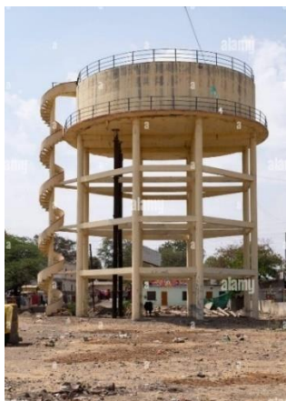
Figure 3: RC frame type Staging
