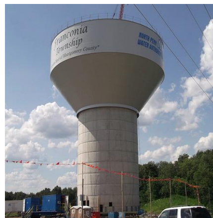
Figure 4: RC shaft type Staging
