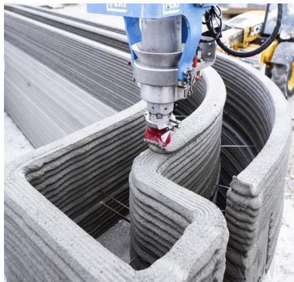
Fig VI : future industry construction
