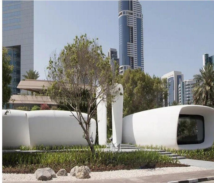
Fig. I V : 3D Printed Office Was Designed For The United Arab Emirates
