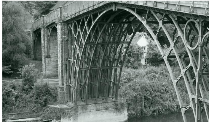
Fig. III The History Of Construction Modu Lac Canada
