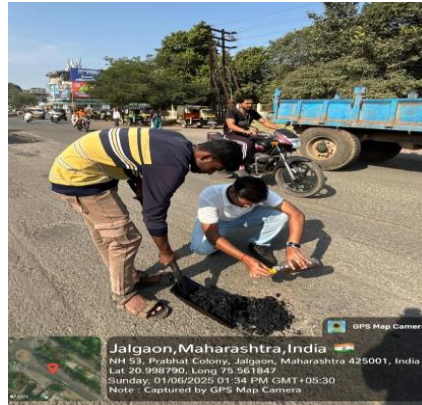
Figure 1: Pothole filling operation.
